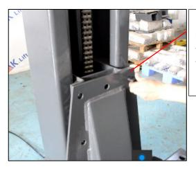
Use forklift to raise the lifting platform to match the mounting hole of carriage and tighten the hex bolts: M20\*40 (with Lock Washer and washer/8pcs)
